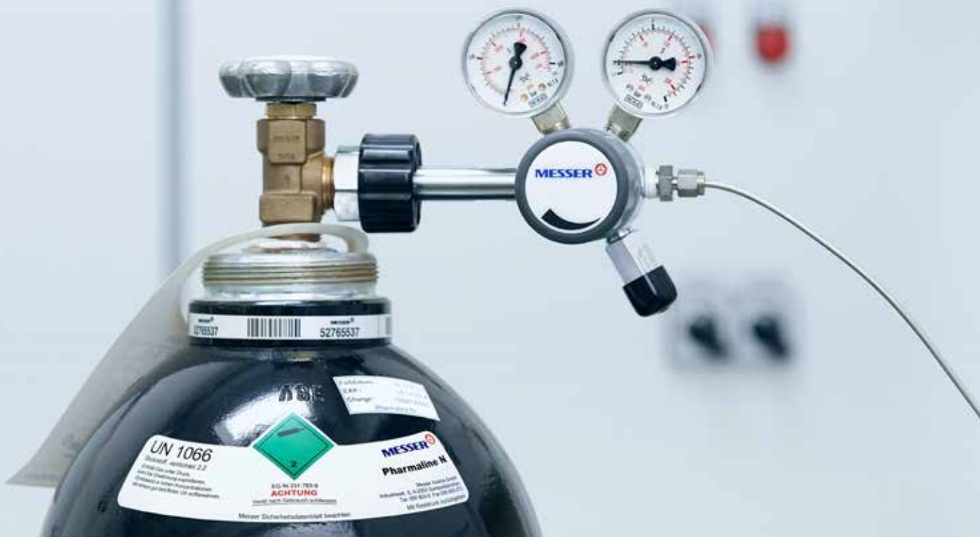
Individual cylinder at the point of use with cylinder pressure regulator
